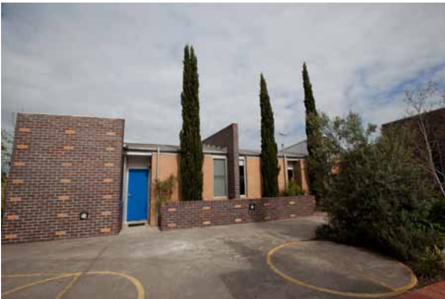
Courtyard at WRAP, showing the semi-detached units
